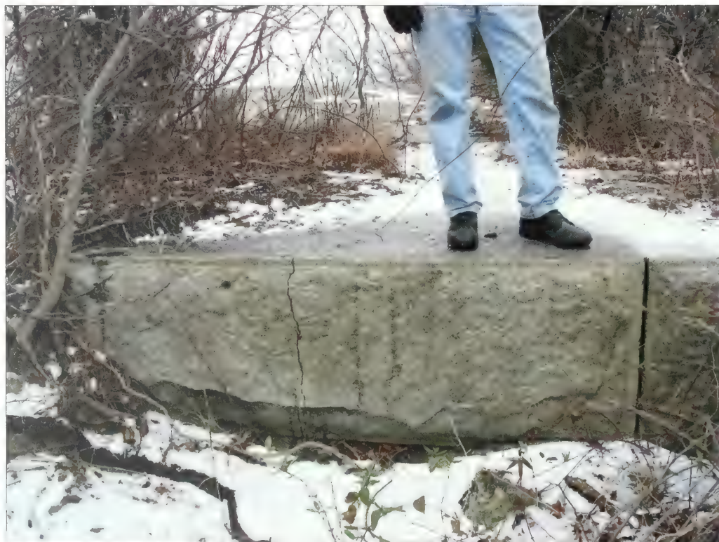
Figure 3.16. Granite blocks northeast of emplacement #8, Nine Gun Battery. Large granite blocks are visible immediately beyond the concrete terreplein. These blocks are remnants of the Civil War-era Fort at Sandy Hook (Olmsted Center, January 2009).
